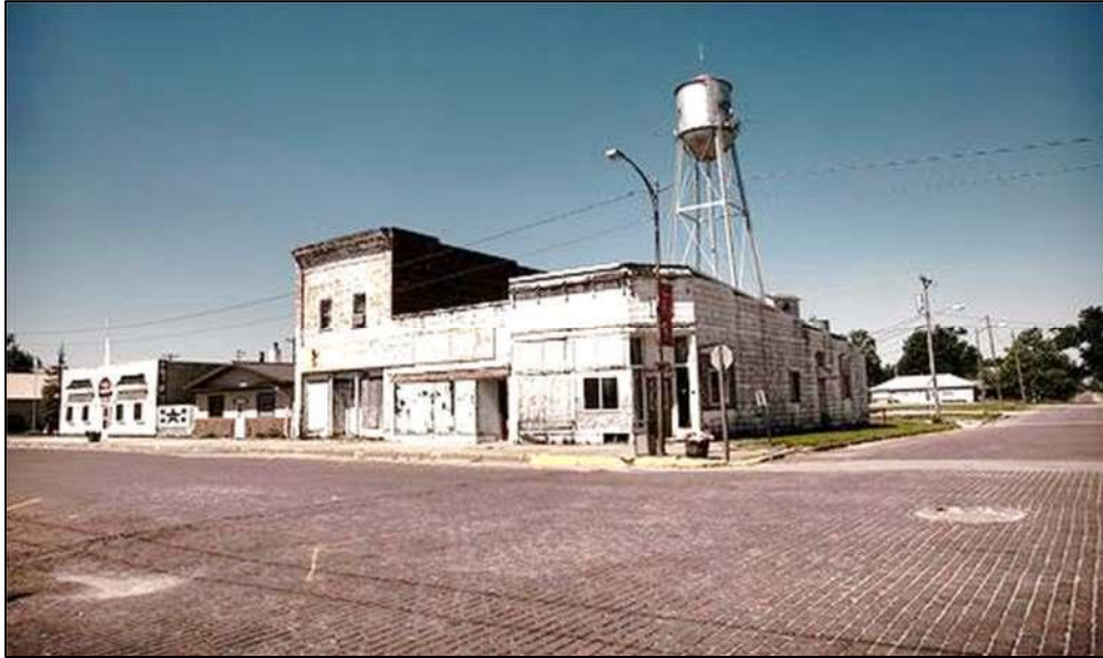
Figure 17. View of water tower behind (west of) the commercial area at the intersection of W 2 nd Street and North Main Street. Note that 2 nd street also has exposed brick pavement as well as Main Street and 1 st Street to the south. Source: Pete Zarria, flickr, accessed at flicker.com and https://www.pinterest.com/pin/369084131936382176/ , accessed June 2022.
