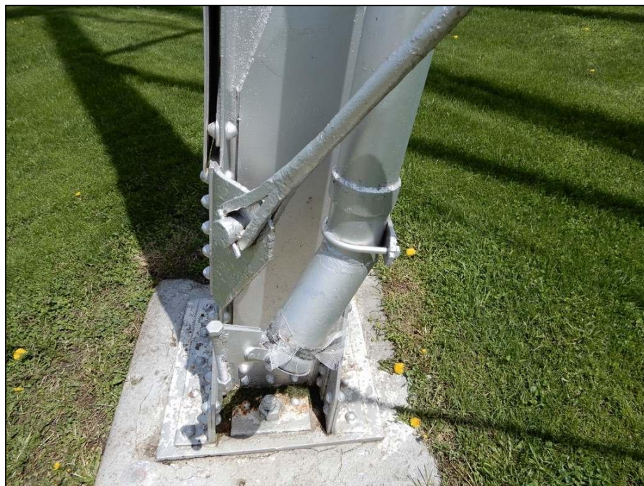
Figure 25. Close up on water tower details. Field date of photograph: May 4, 2022.
