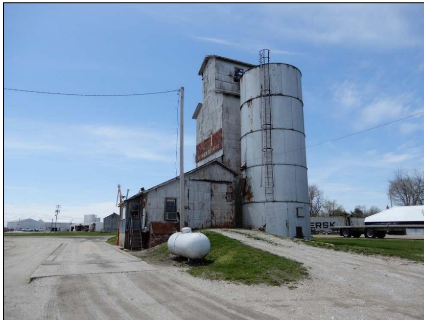
Figure 16. Facing SW towards Hedrick elevator. Field date of photograph: May 4, 2022.
