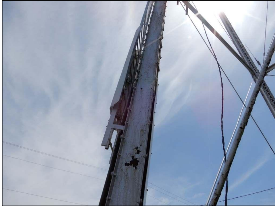
Figure 22. Close up on water tower details. Field date of photograph: May 4, 2022.
