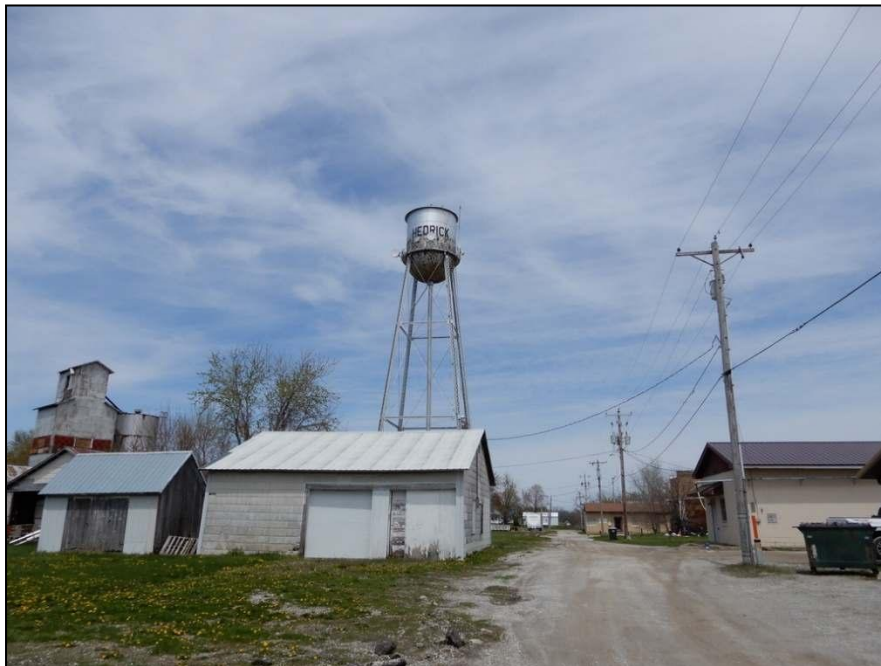
Figure 10. Facing north towards water tower and surrounding buildings. Field date of photograph: May 4, 2022.
