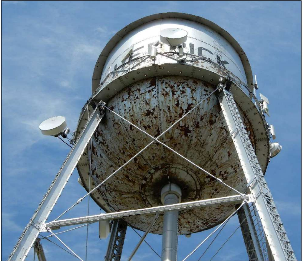
Figure 32. Close-up of base of water tank showing legs, webbing, zig-zag railing and the many communication devices since added to that railing.
