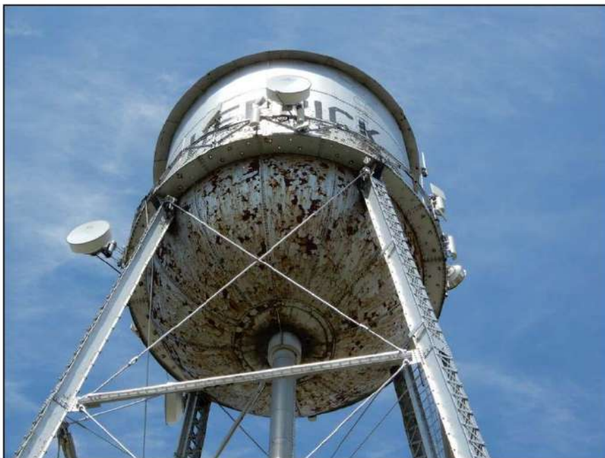
Figure 20. Close-up on base of water tank showing general condition. Field date of photograph: May 4, 2022.
