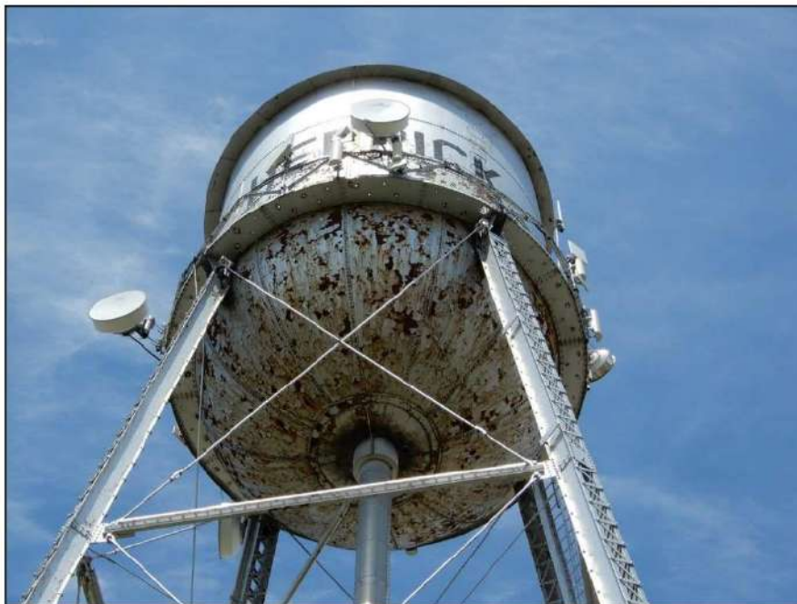
Figure 29. Close up on base of water tank showing general condition. Field date of photograph: May 4, 2022.
