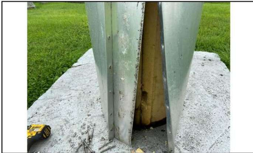
Figure 37. Metal wrapping of insulation on vertical pipe. Source: Viking Industrial Painting 2020:E3.
