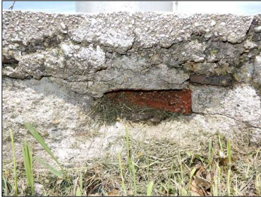
Figure 30. Close up on cement foundation at center of water tower and brick embedded within. Field date of photograph: May 4, 2022.
