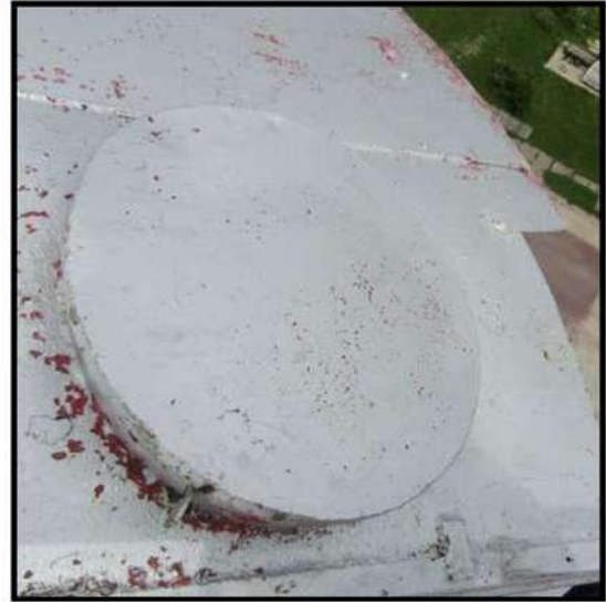
Figure 36. Close-up view of cylindrical roof vent that may have replaced the original cast iron finial and the roof manway, looking west. Source: Viking Industrial Painting 2020:9-10.
