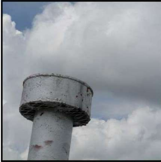
Figure 36. Close-up view of cylindrical roof vent that may have replaced the original cast iron finial and the roof manway, looking west. Source: Viking Industrial Painting 2020:9-10.
