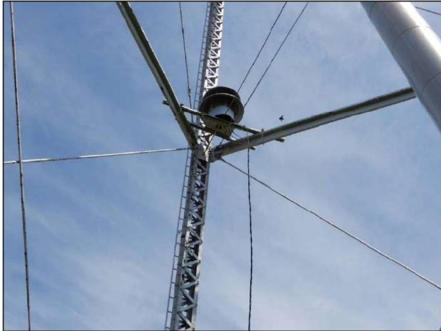
Figure 28. General view of water tower joint details and city siren. Field date of photograph: May 4, 2022.
