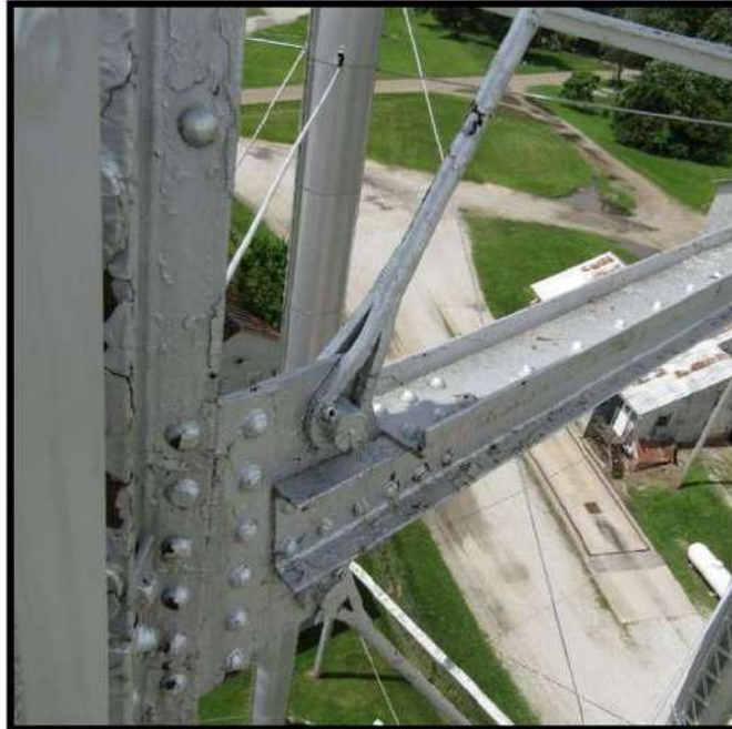
Figure 34. Northeast leg, looking south. Upper strut joint with angled rod and leg. Source: Viking Industrial Painting 2020:5.
