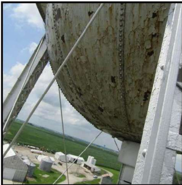
Figure 35. Close-up view of belly and balcony with safety cable, looking west. Source: Viking Industrial Painting 2020:6.
